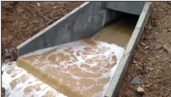
Scroll over picture and click to activate video and watch the headwall in action
